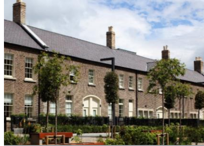
Multifamily : Clancy Quay, Dublin, Ireland
