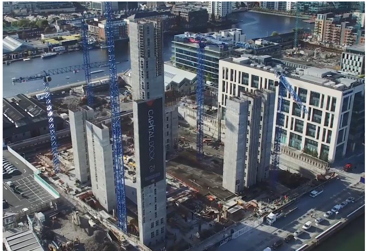
Construction in progress at Capital Dock, Dublin
