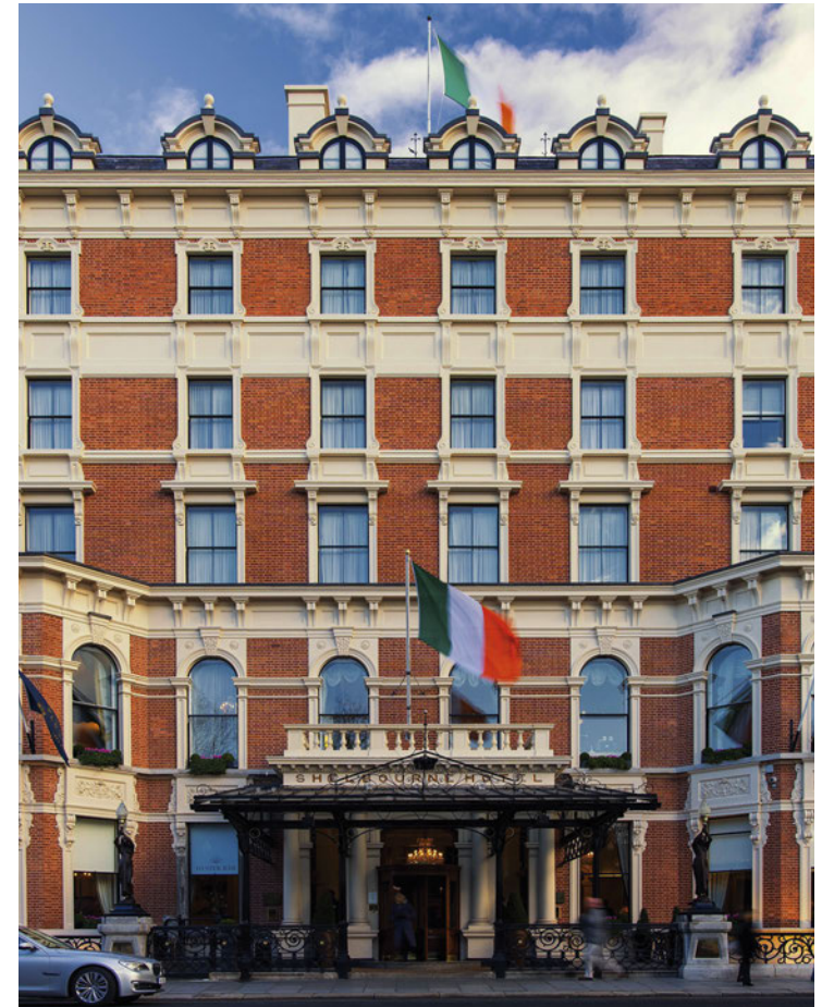
Shelbourne Hotel Dublin, Ireland
