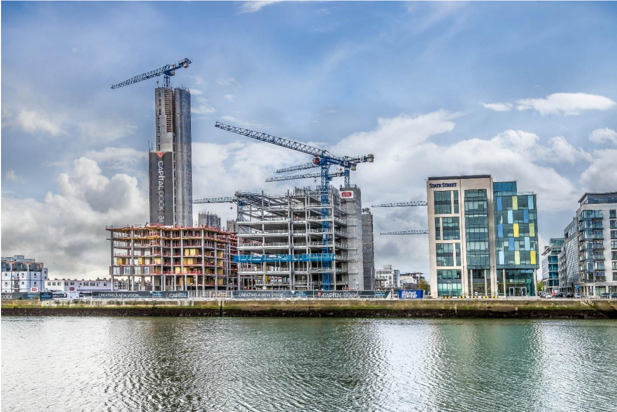
Construction in progress at Capital Dock (Dublin, Ireland)
