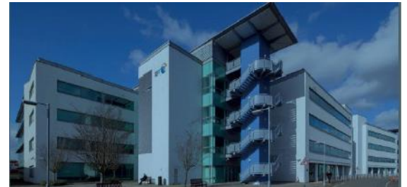
South East Office
